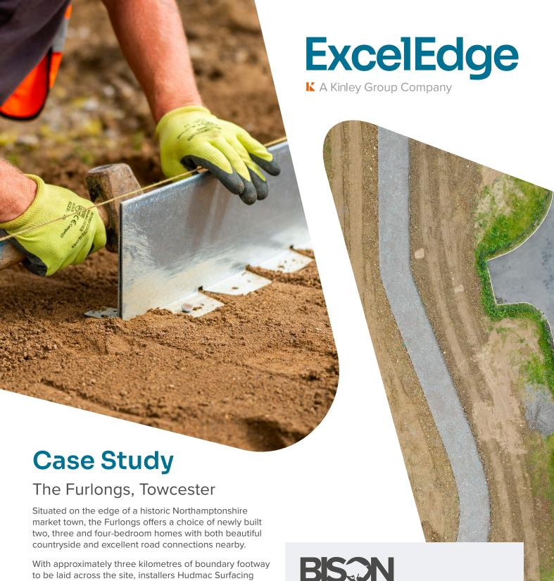
wanted an edging product that is quick and easy to install, but at the same time more durable than timber and less prone to cracking than concrete.
