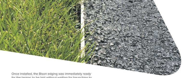
for the tarmac to be laid without waiting for haunching to cure, as is the case with concrete edging.
